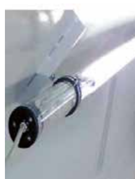
ATEX special lighting
